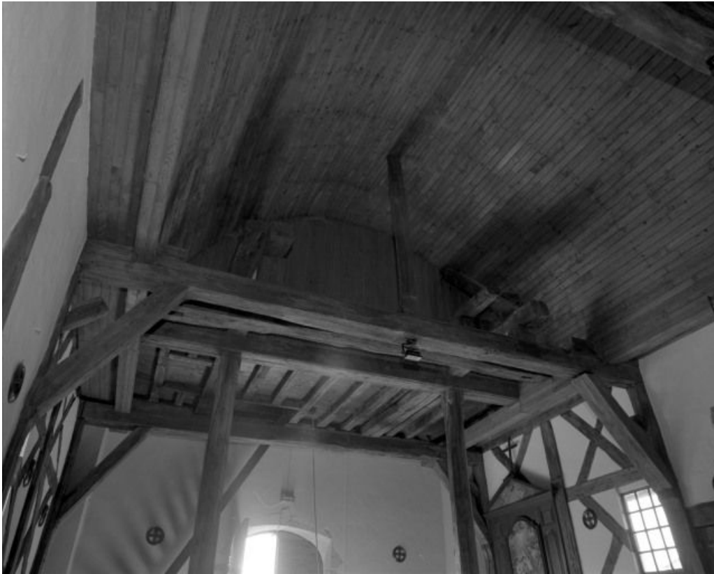
Nef, charpente soutenant le clocher.
