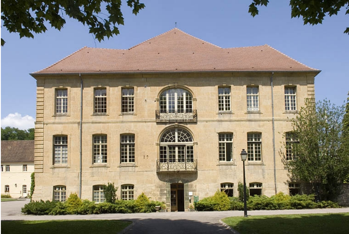
Logis abbatial. Façade sud.
