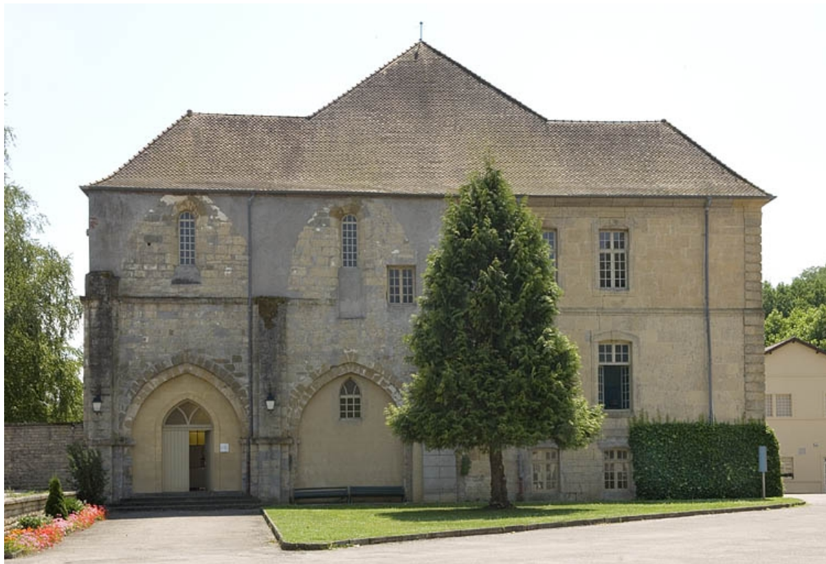
Logis abbatial. Façade nord.
