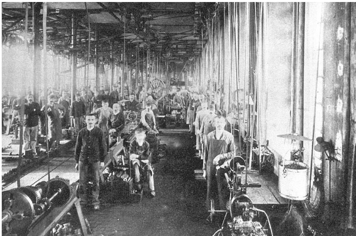
Atelier de construction.
