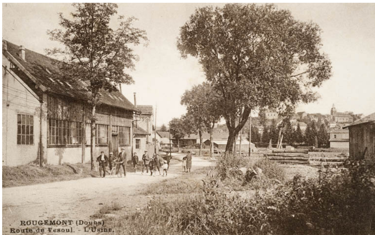
Rougemont (Doubs). Route de Vesoul-L'Usine.
