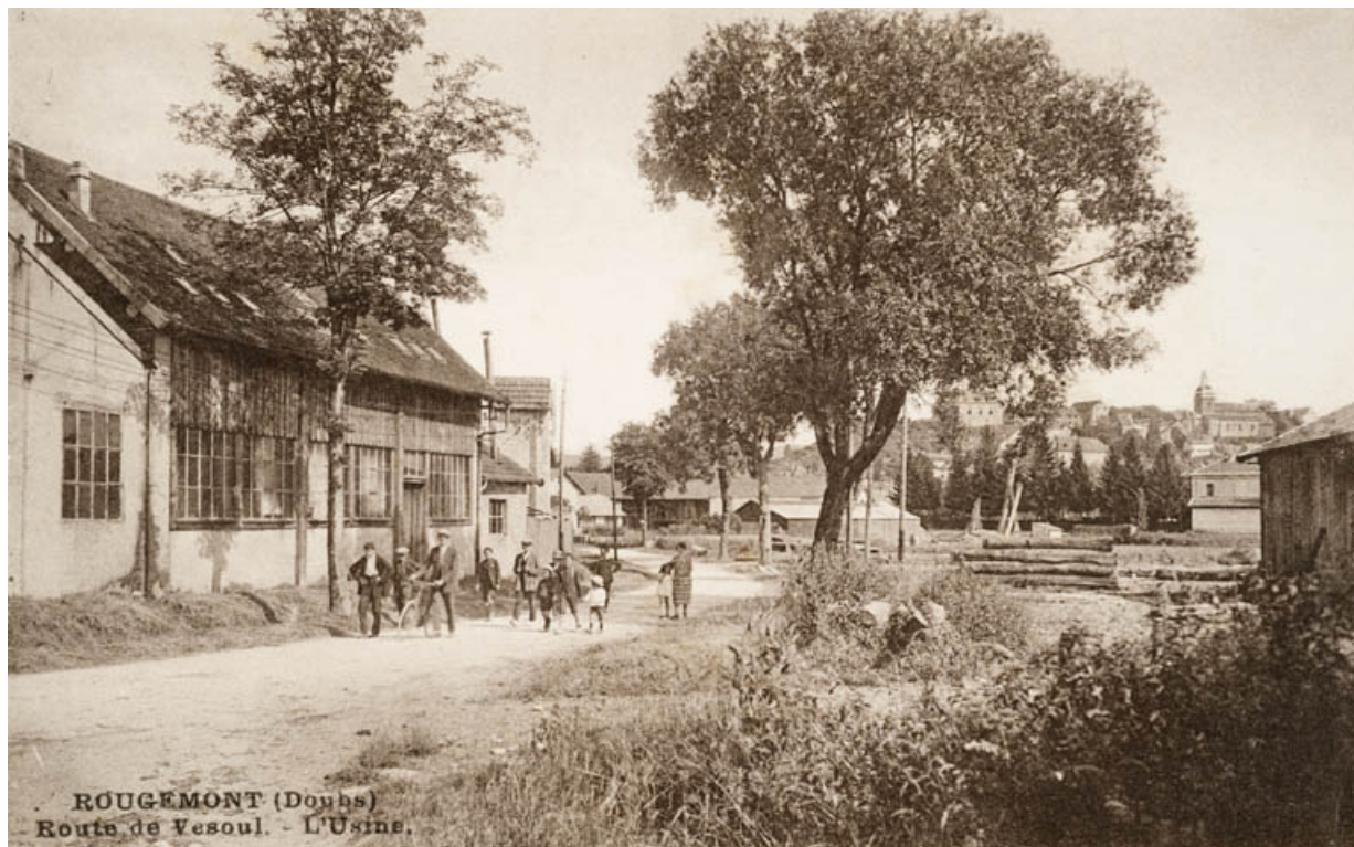
Rougemont (Doubs). Route de Vesoul-L'Usine.
