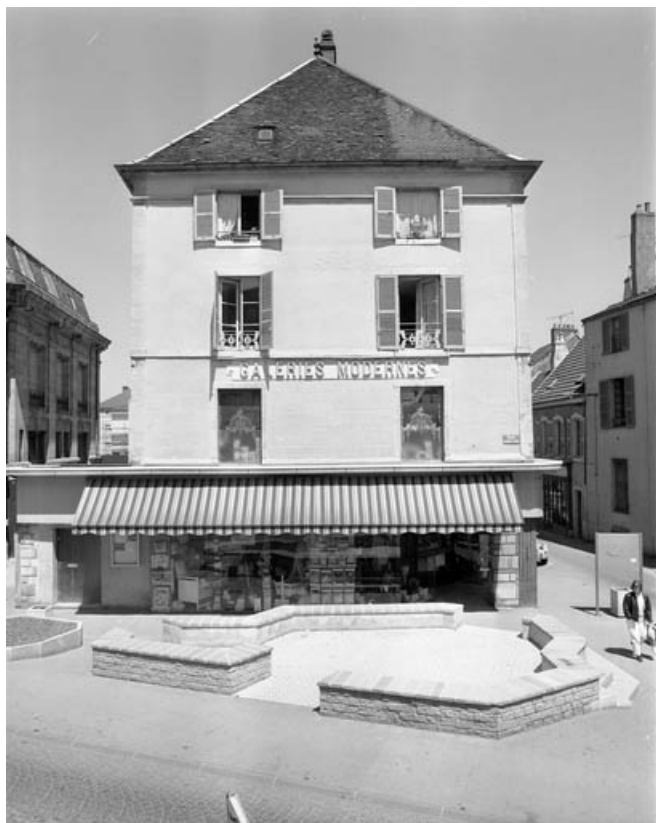
Façade principale, de face. 70, Gray place Bour Edmond
