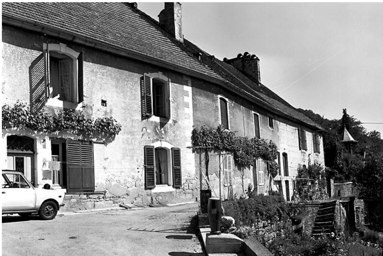
Façade antérieure. 25, Lods
