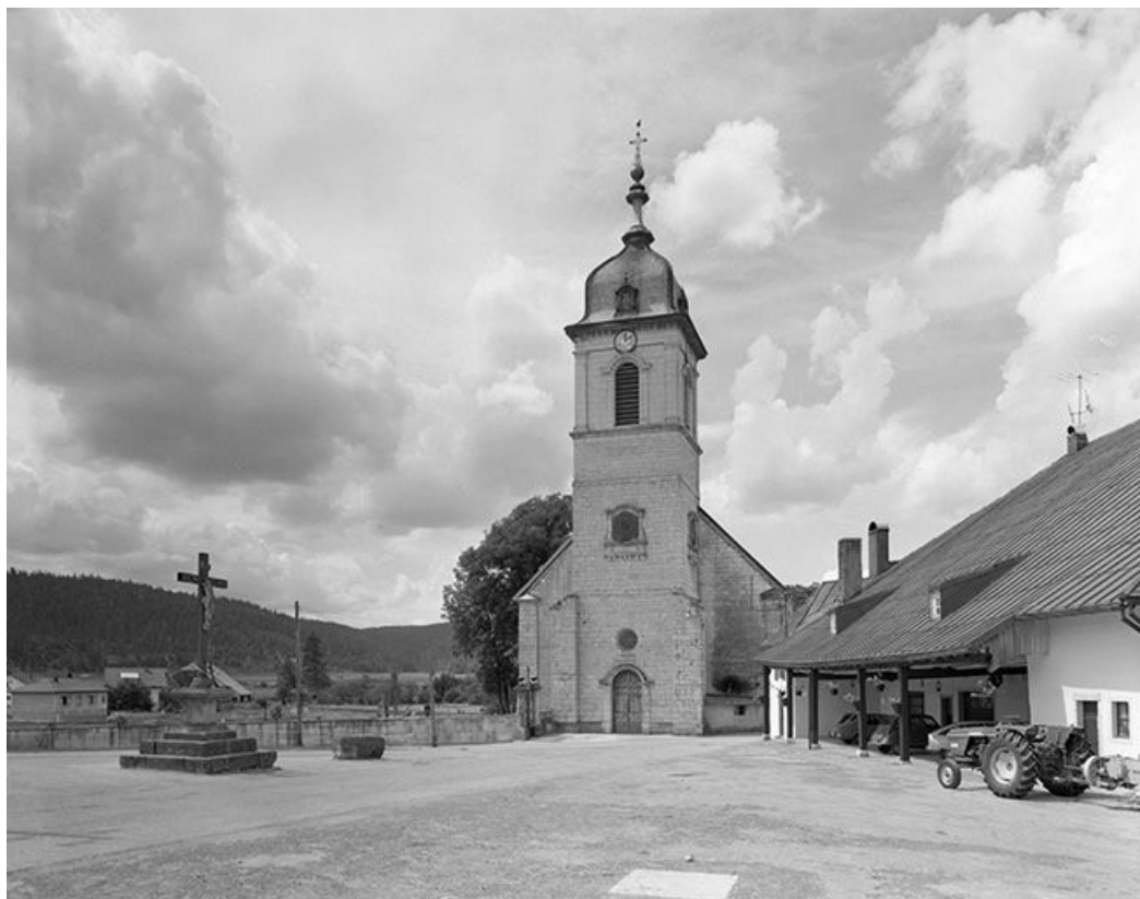
Façade antérieure. 25, Mouthe
