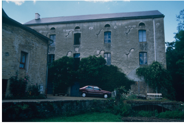
Elévation sud. Phot. Delarozière Benoit, Phot. Delarozière Olivier IVR26_20058900087ZA
