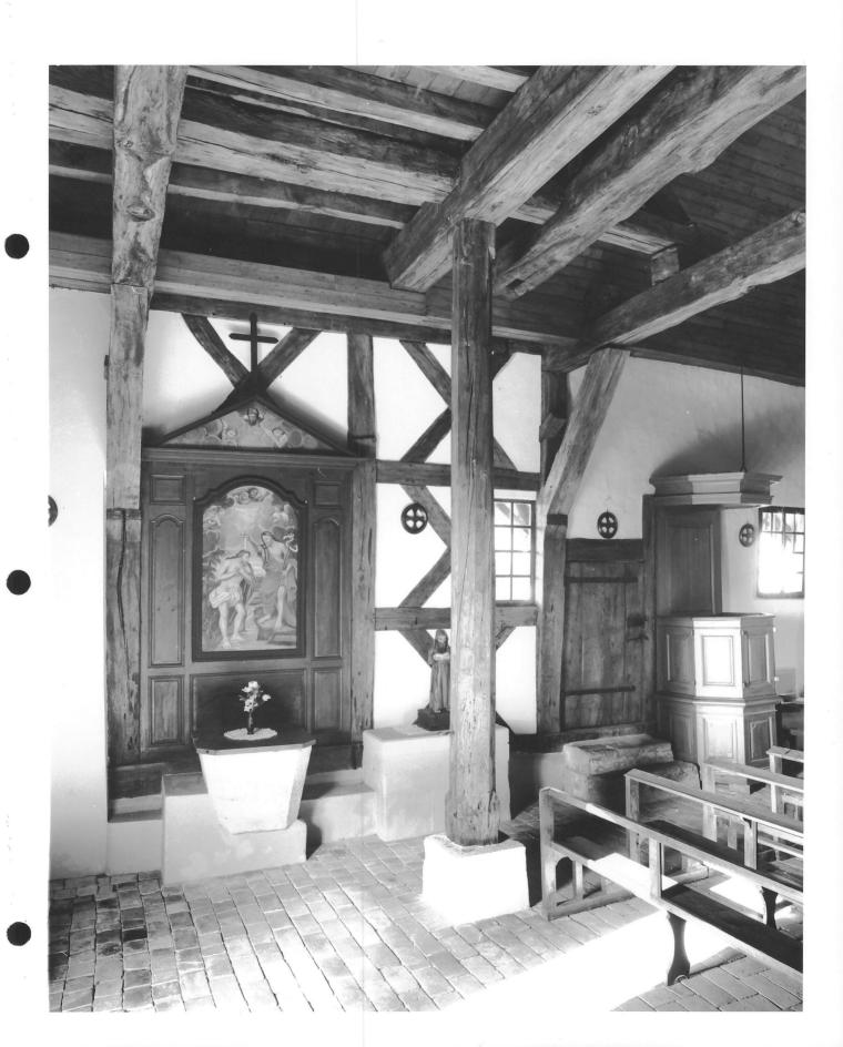
Fig. 12 Nef, charpente soutenant le clocher.
