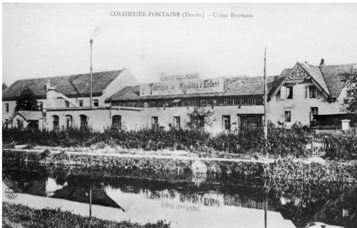
Colombier-Fontaine (Doubs). Usine Baumann.
