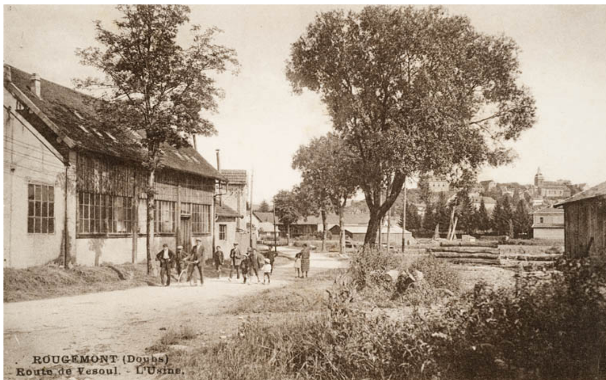
Rougemont (Doubs). Route de Vesoul-L'Usine.
