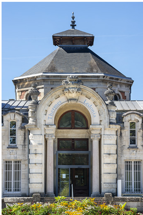
Façade principale, portail.
