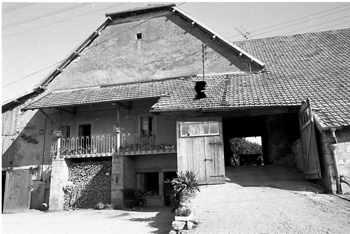
Façade antérieure. 25, Tarcenay
