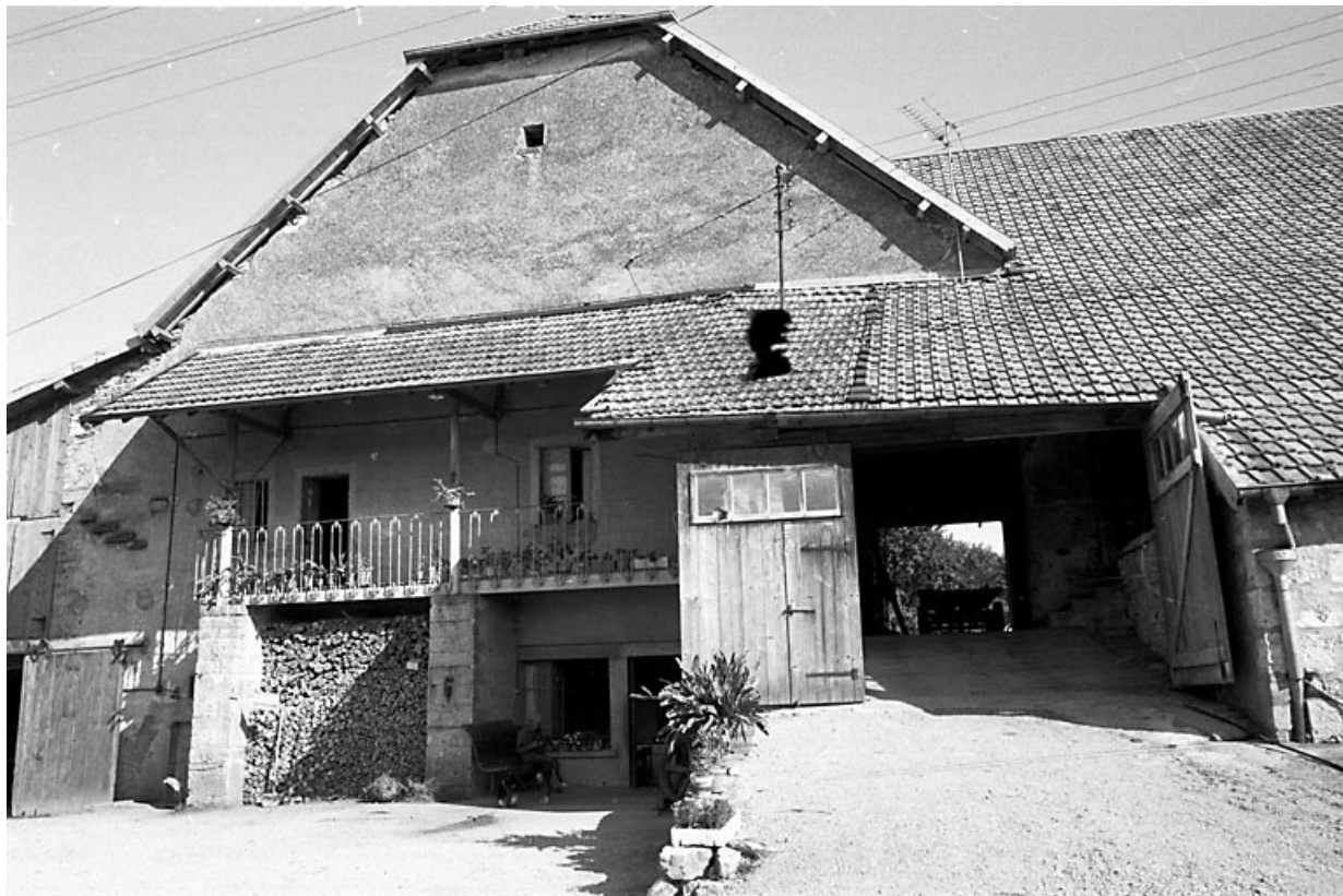
Façade antérieure. 25, Tarcenay
